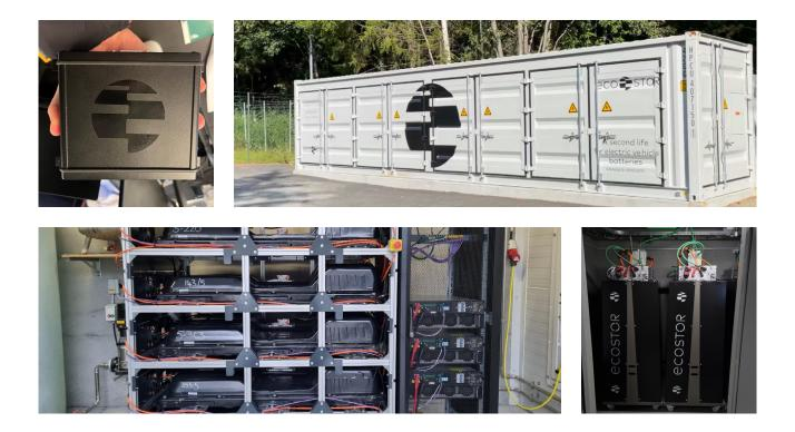
The picture at the bottom left shows the batteries without the case. On the far right, the inverters can be seen.
